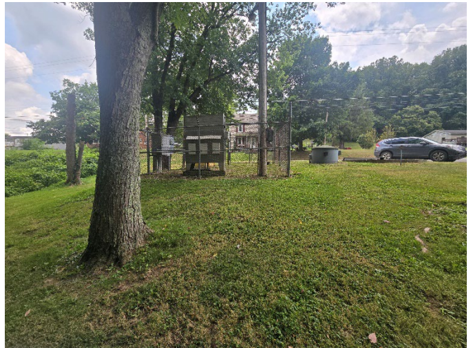
8. Pump B6 – Facing East
