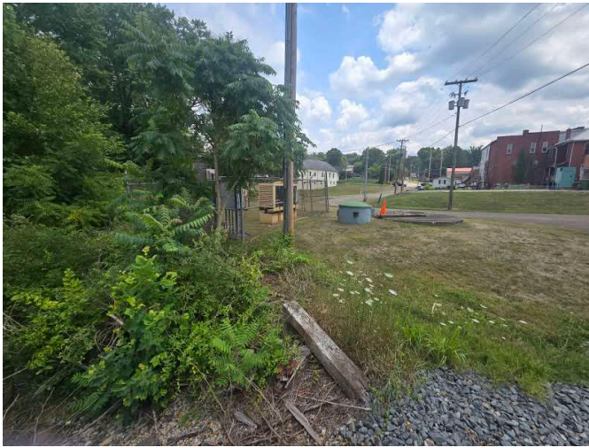
1. Pump B1 – Facing East
