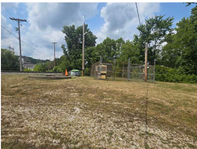
5. Pump B1 – Facing West
