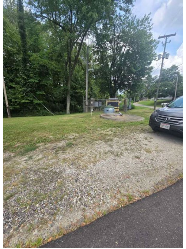
14. Pump Station 6 – Facing North from Mohican Road.
