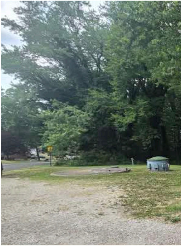
13. Pump Station B6 – Facing North – Close Up
